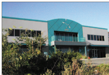
PRBO's new San Francisco Bay Research Center and Headquarters. PRBO photo
